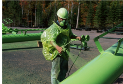
Custom color on Metal Pipeline Airless
