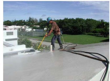
Concrete roof application 25,000 Sq ft area
