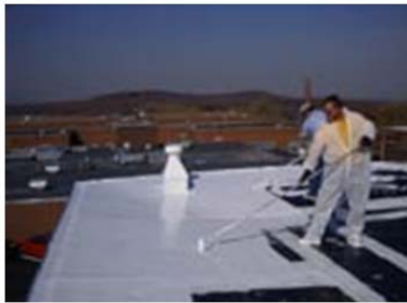
Application over Firestone EPDM
