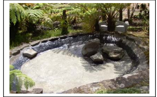
Perimeter coated with Liquid Rubber
